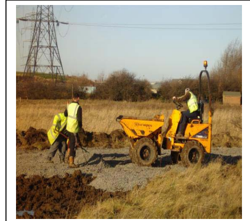
Backfilling with blast furnace slag
